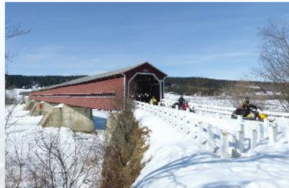
Covered bridge at Notre-Dame-des-Pain.
